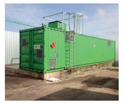
MOBILTANK® ISO is a compact, robust, movable and autonomous station allowing the remote management. This mobile station designed from sea shipping container, integrates the highest security standards. Our MOBILTANK® are also customizable depending on your needs: loading arm, filling pump, power generator...
